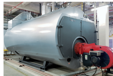
Vitomax HS (13,0 t/h, 10 bar) Cliente: PT. B. Braun Pharmaceutical Indonesia
